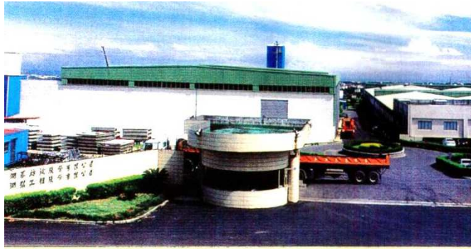
The No. 9 Plant
